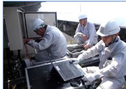
■ Inspection service for solar power plants
